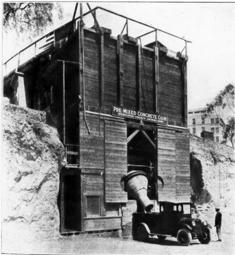
The Pre-Mixing Concrete Plant
